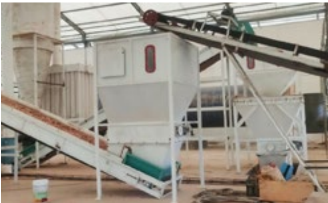
Biofuel Manufacturing Plant
